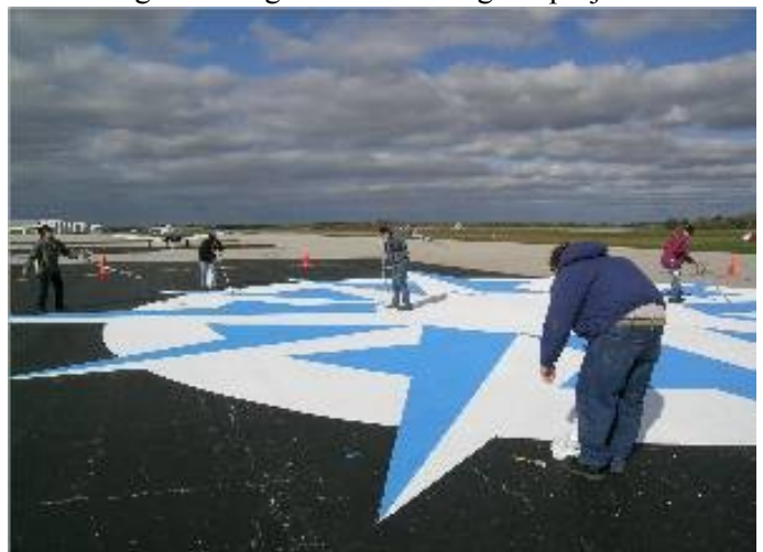
Painting's done. Time to remove the masking tape.
